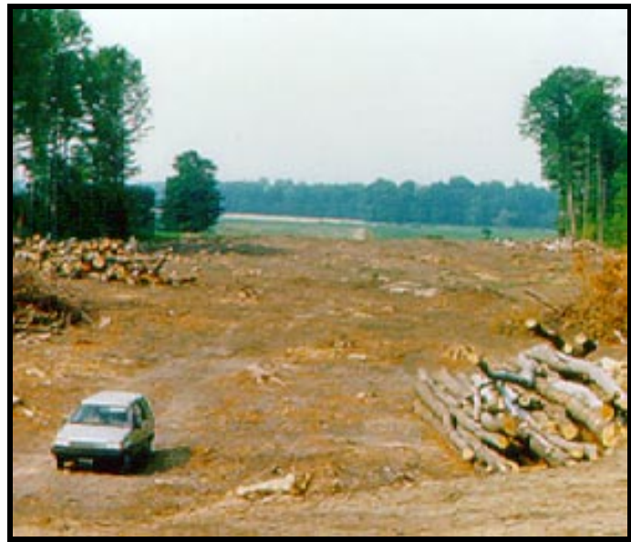
Figure 14 The Beachridge Site After ROW Preparation.
